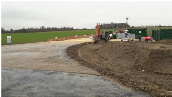
Wind farm access bell-mouth looking east from edge of A1 northbound
