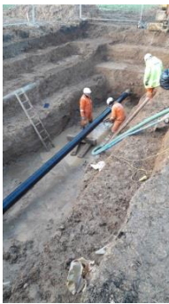
Oil pipe re-wrapping
